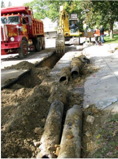
Water Main Replacement Construction
