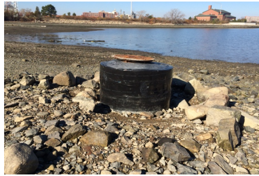
Sewer Manhole at Beach - Raised and Sealed
