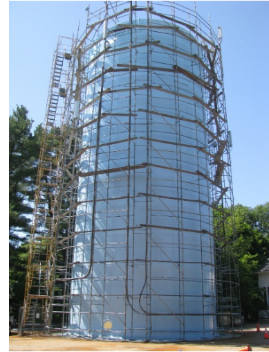
Rehabilitated Water Storage Tank
